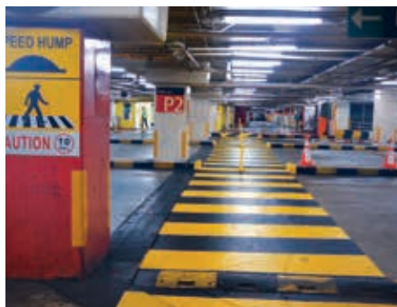
Speed humps and pedestrian crossings are placed at strategic locations within the KLCC's North-West Development car park for customers' safety.
